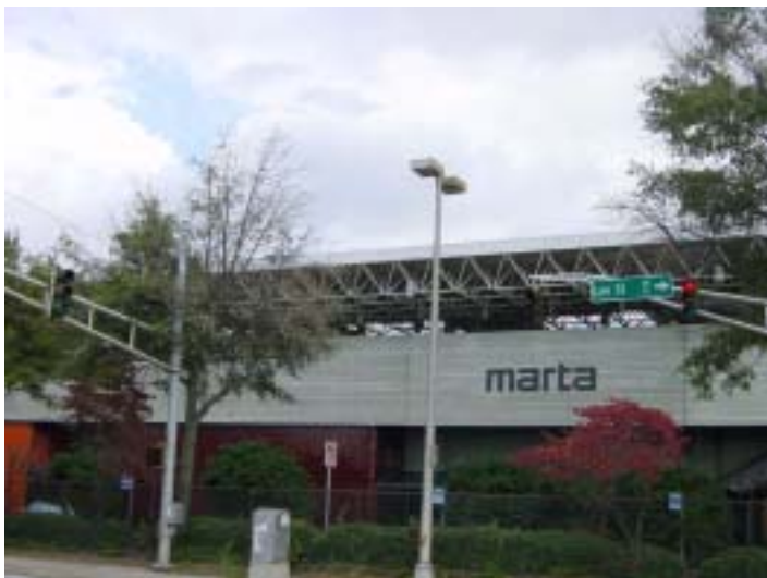
The area surrounding the West End MARTA station will incorporate smart growth strategies to encourage commercial development and sustain the historic integrity of the West End Historic District. Photo by Jeanne Cyriaque
